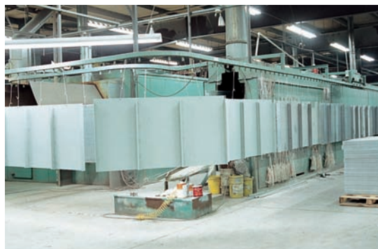
The powder coating process begins and ends at this point: parts travel by conveyor through a 5-step cleaning process, the FoxGard spray booth and finally the curing oven.
